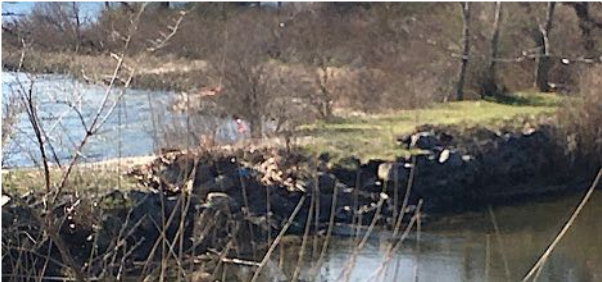
ABOVE: Photo of the pedestrian causeway marked on the aerial above as at "A".
