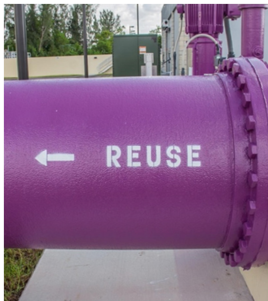
Figure 2 - Purple pipes carrying reclaimed water in Florida
