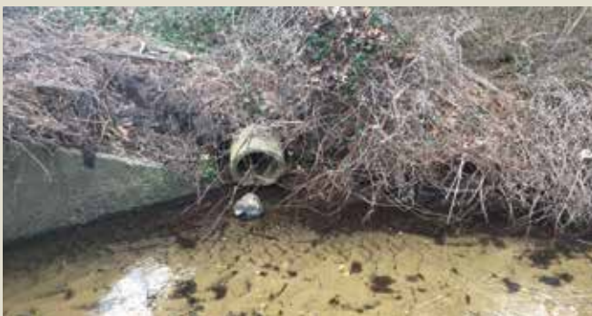
Storm Water Discharge
